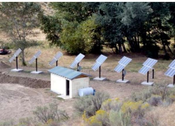
pump is used to pressurize the drip irrigation on 30 acres of 2-month-old vines, with an additional lift of 20ft.
